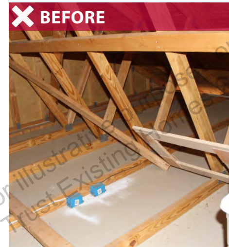
Attic without insulation
