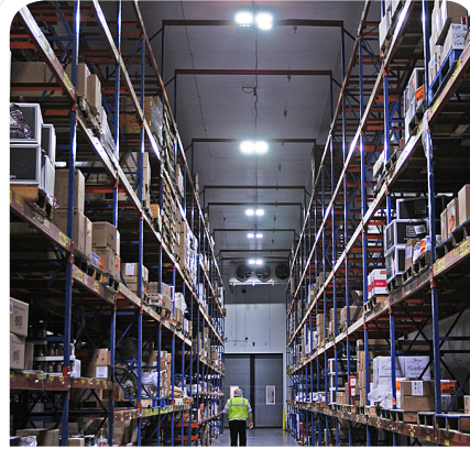
LED high-bay lighting provides even illumination throughout the warehouse and controls turn the lights off when the space is not in use
