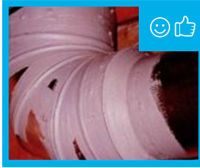
Fig. 33: Mastic is nickel thick and covers both connections and gores to ensure a tight seal.
