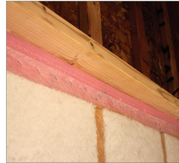
Fig. 7: Foam sill sealer installed at top plate
