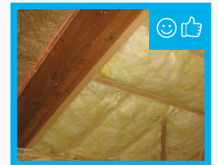
Fig. 25: Insulation is friction-fit, has no gaps or cracks, and fills the cavity.
