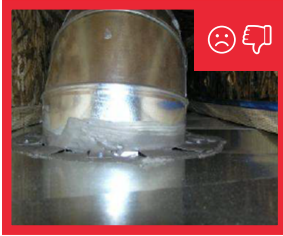
Fig. 32: Duct sealing mastic was used too thinly and does not fill the holes.
