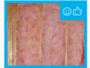
Fig. 23: Well-fit insulation, filling the cavity, with no gaps or cracks.
