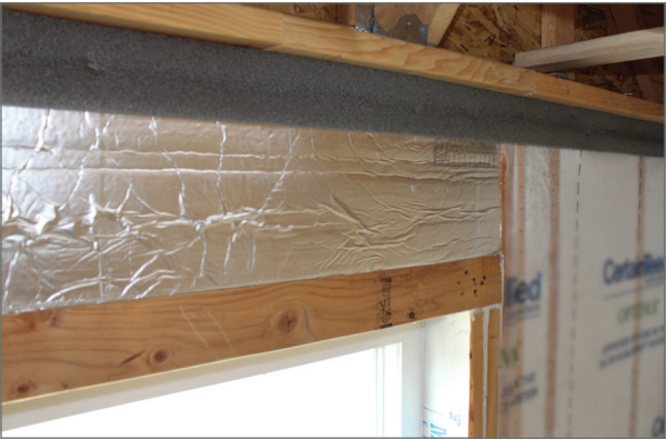
Fig. 4: Insulated header
