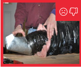
Fig. 30: Mechanical seal (Panduit strap or zip tie) is not connecting flexible duct to metal boot.
