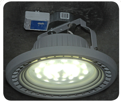
PHOTOS LEFT TO RIGHT: Daylighting and photo sensors with linear fluorescent; LED with wireless control
