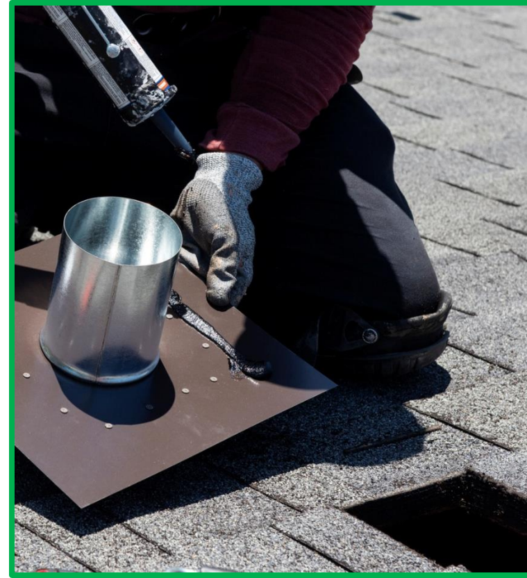
ILLUSTRATION AT 1.6-EXHAUST BOOT CONNECTED TO SHEATHING
