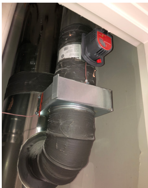
• Programmable supply interconnected with exhaust fan (1.0 sones or less)
