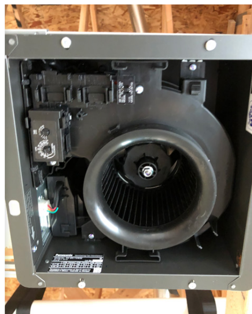
• Programmable supply interconnected with exhaust fan (1.0 sones or less)
