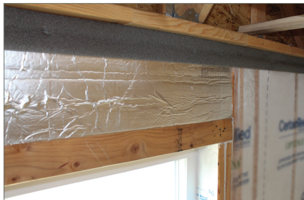
Fig. 4: Insulated header
