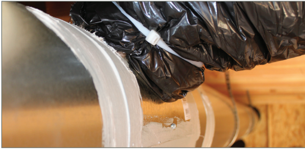
Fig. 28: Nickel-thick mastic
