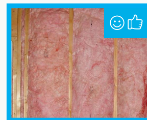
Fig. 23: Well-fit insulation, filling the cavity, with no gaps or cracks.
