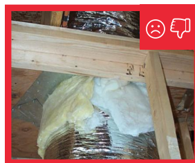
Fig. 10: Penetrations around duct using fibrous insulation do not seal the attic against air movement to the chase.
