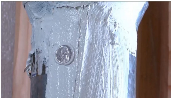
Fig. 28: Nickel-thick mastic
