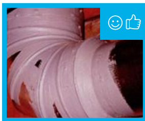
Fig. 33: Mastic is nickel thick and covers both connections and goes to ensure a tight seal.
