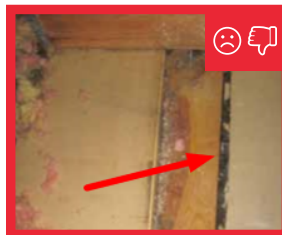
Fig. 12: Top plate is not air sealed, connecting attic air to interior wall.
